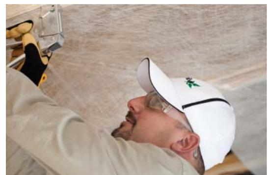
4. Taking a straight, factory netting edge, the crew may either start stapling across the peak or down the eave, stretching the netting tight along the stapled edge.
