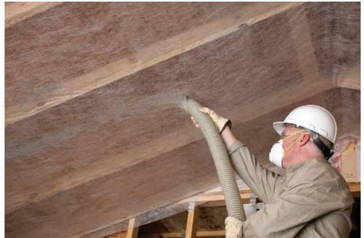
4. The time to fill a cavity will depend on the machine being used, the material flow and air settings. The material should not clog the hose during this process. If the hose does clog, clean out the hose and close down the feed gate by 10% or increase the air flow until clogging does not occur.
