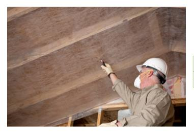
3. Begin filling cavity; do not allow the material flow to back the hose up the cavity on its own. Create some resistance in order to ensure full cavity density. Slowly retract the hose in order to avoid clogging the hose. Ensure that the Dry Dense-Packing at the ridge is complete to avoid the potential for settling.
