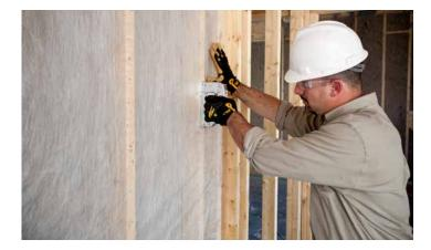
6. Complete the wall by stapling the bottom edge of the netting across the length of the bottom plate.
