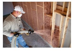
Only Greenfiber FRM Insulation may be used as a fireblocking material in the the SANCTUARY Two-Hour Firewall, UL-U370 assembly. This product can be identified by it's proprietary a terracotta color.
