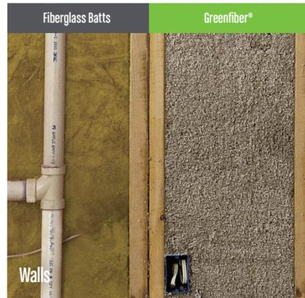
Greenfiber cellulose insulation fills cavities from side-to-side and top-to-bottom, without gaps or voids around obstructions like blocking or bridging, and it fits tightly around wiring or electrical boxes within the cavity for a Grade-1 install that blocks sound and resists air infiltration.
